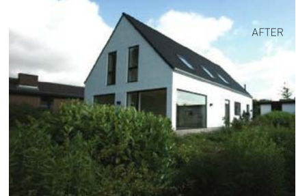
A house from the seventies was totally redesigned and made to fit a modern family of five.
